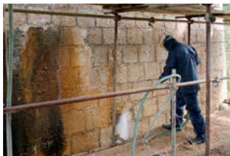
Cleaning building scaffolding
