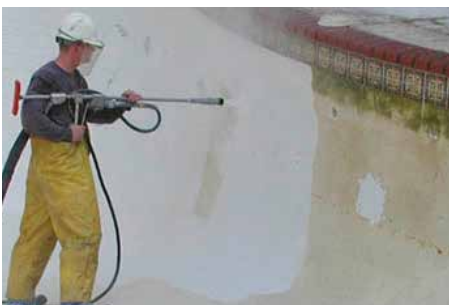
Removal of paint, rust and graffiti from steel and/or concrete surfaces
