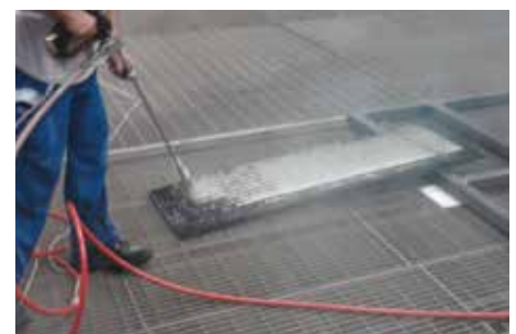
Hydrosandblasting
